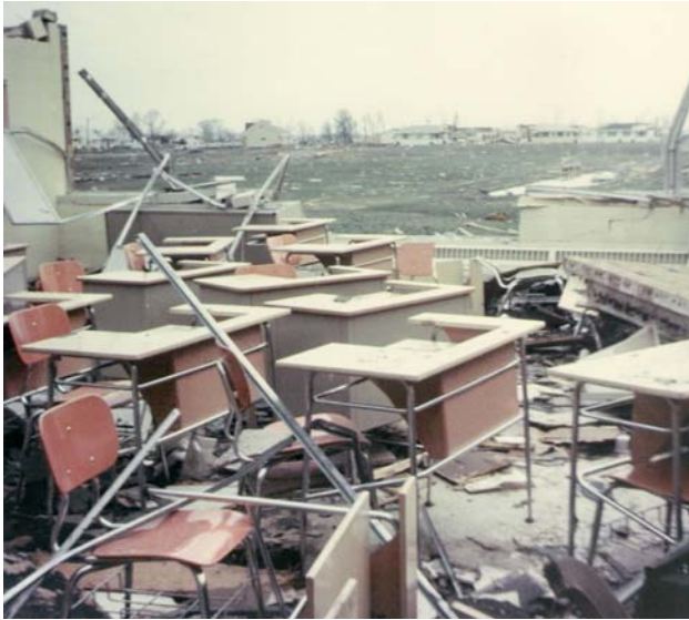
Damage from the May 6, 1965 tornado.
