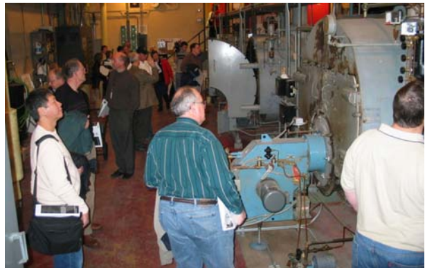
Task Force members view a 50-year-old boiler during a tour of the high school complex
